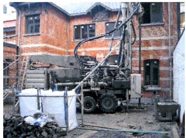
Drilling in the courtyard of the REH
