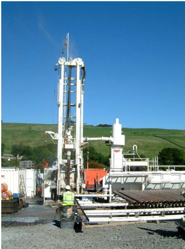
FORACO rig at Eastgate
