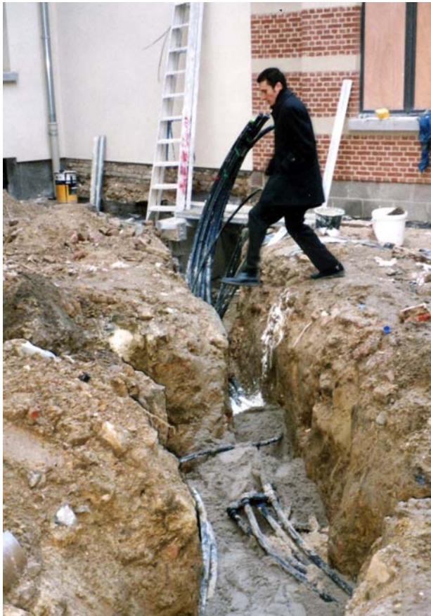
Philippe Dumas crossing the collector pipe trenches
